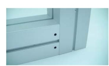
When the lock is properly engaged, the extrusions will fit tightly together.
